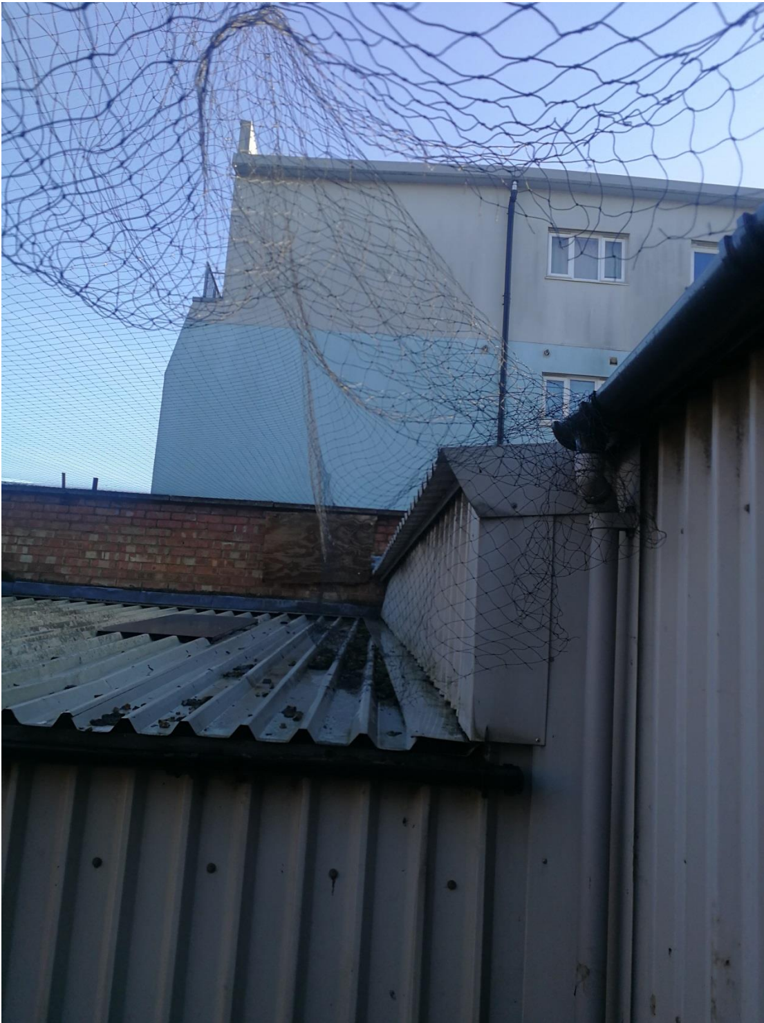
Side elevation of Birchfield
